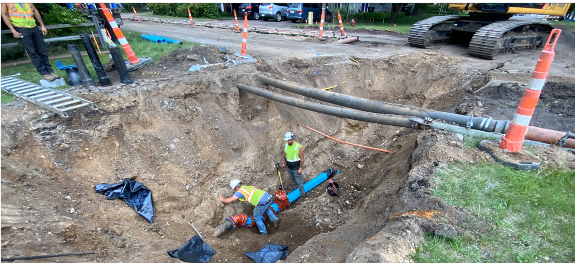
The Contractor installs new watermain and gate valves at the intersection of 1st Street and Char Avenue
